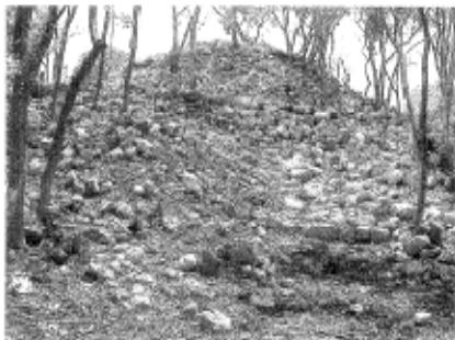
Fig. 5. The Cave Pyramid looking west after preliminary clearing. This Pyramid is directly above the cave and shows Megalithic stonework and staircases similar to Middle Preclassic architecture recently identified at nearby sites such as Xocnuc.
